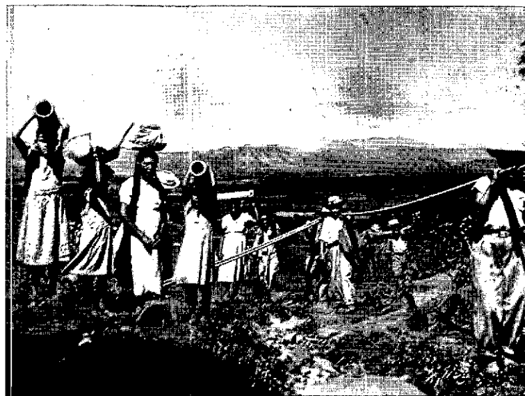
The people of a rural town take an active part in laying the pipes for their new water supply.
